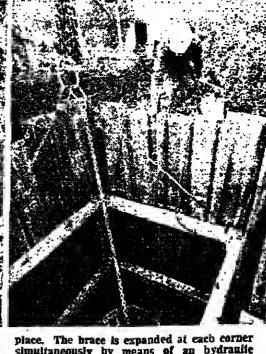
simultaneously by means of an bydraulie pump. If the excavation is not square, the brace will automatically adjust to provide equal support at each pnint.
